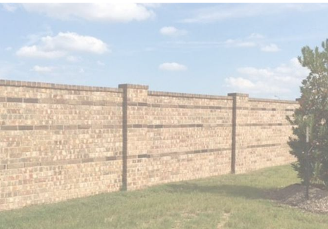
MASONRY WALL BRICK COLOR AESTHETIC
