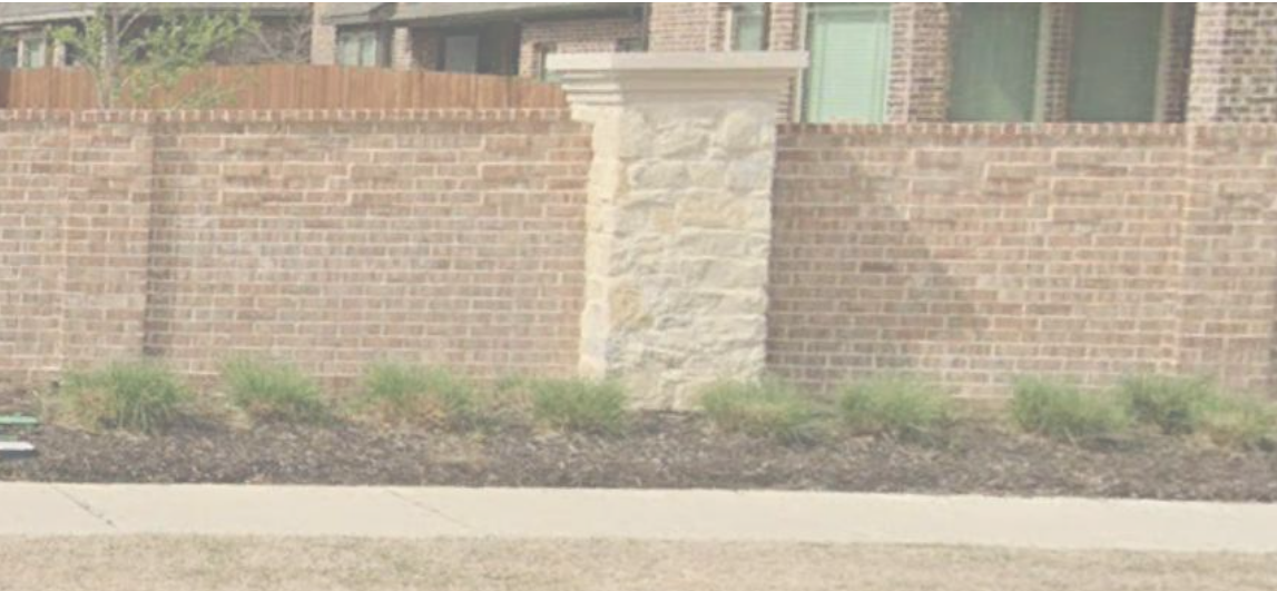
MASONRY WALL COLUMN AESTHETIC
