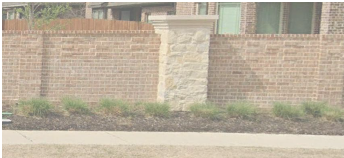
MASONRY WALL COLUMN AESTHETIC
