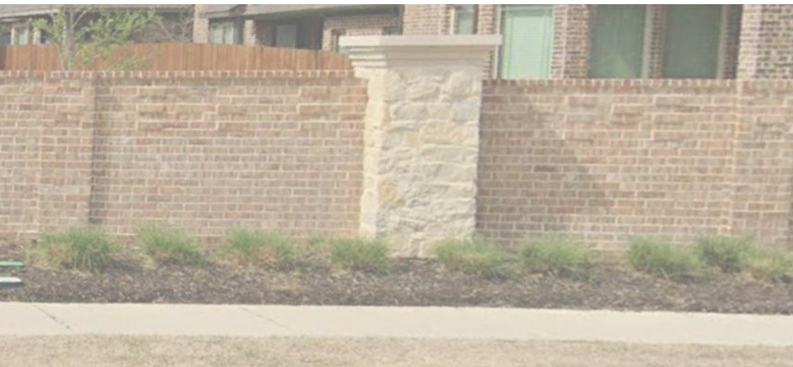
MASONRY WALL COLUMN AESTHETIC
