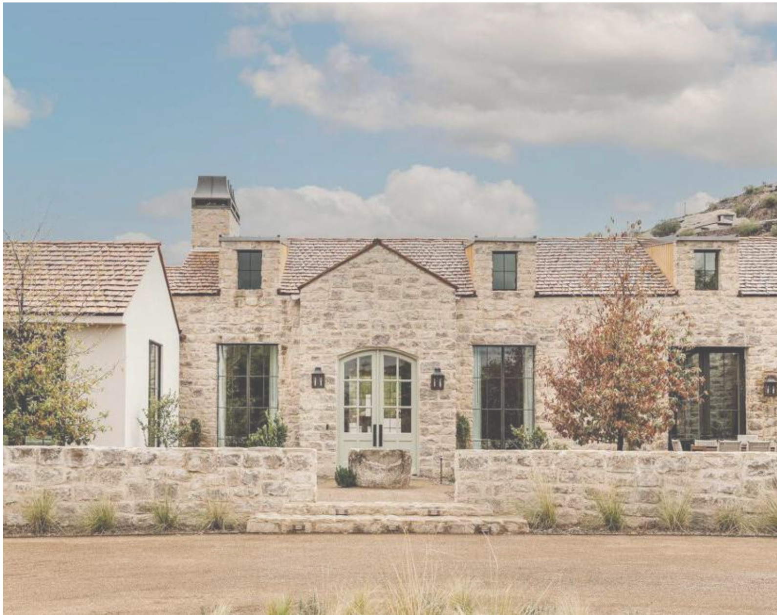
ARCHITECTURAL AESTHETIC - AMENITY CENTER
