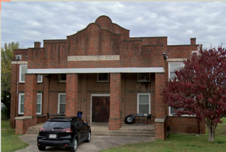
MISSION Curvilinear parapets, overhanging eaves with exposed rafter tails, and deep, simple shapes, reflecting a blend of simplicity and grandeur.
