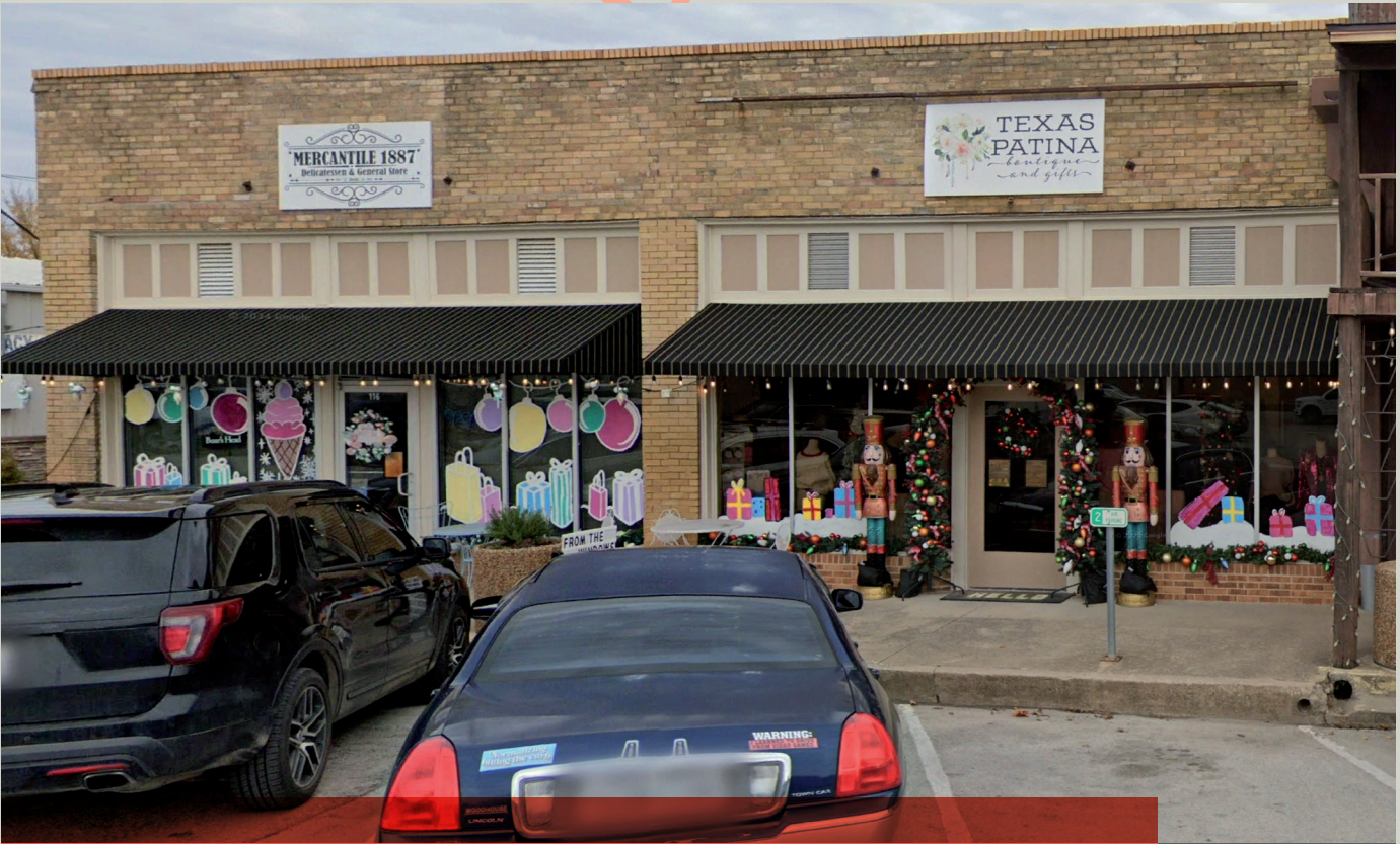
REGARDLESS OF THE DIFFERENT ARCHITECTURAL STYLES AND TIME PERIODS, THERE ARE CONSISTENT ELEMENTS ALONG 4TH STREET SUCH AS BUILDING PLACEMENT AND AWNINGS. 4TH STREET
